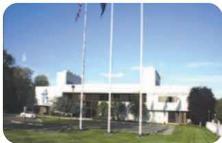
Southern Connecticut Gas Utility - USA
