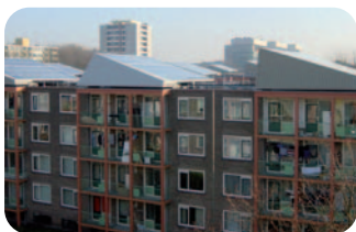
MFH 2 MW Project - Netherlands
